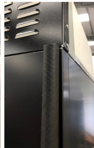
Align back spacer with back edge of cabinet and vented pelmet
