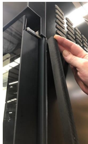
Align front spacer with plastic door frame and bottom of vented pelmet
